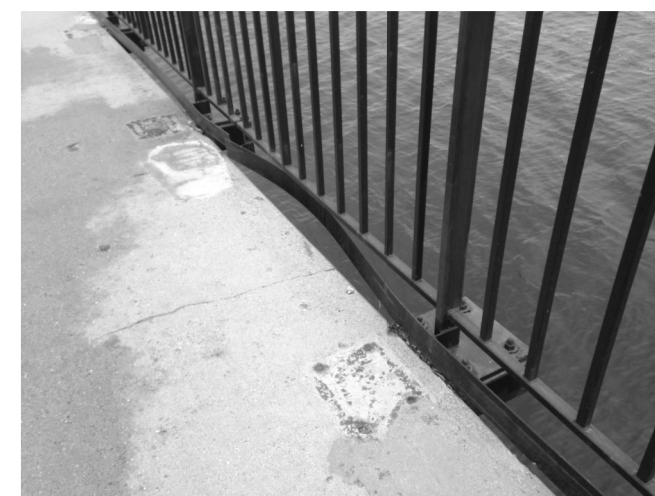
TYPICAL BENT TOE BOARD
